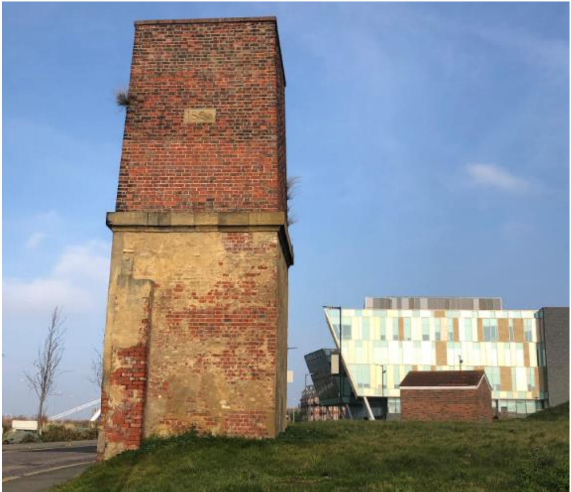
Figure 6.2 Swinburne Glassworks Chimney
